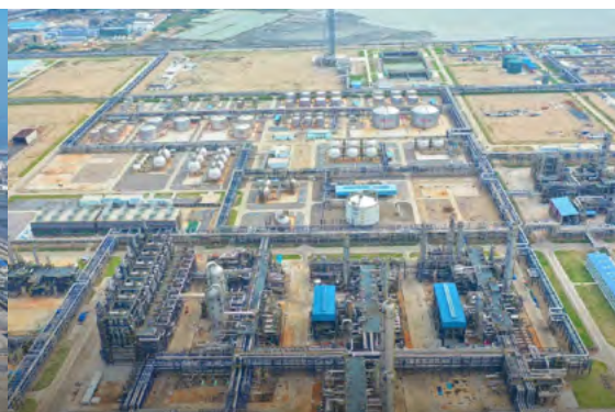
Aerial view of the steam cracking unit
