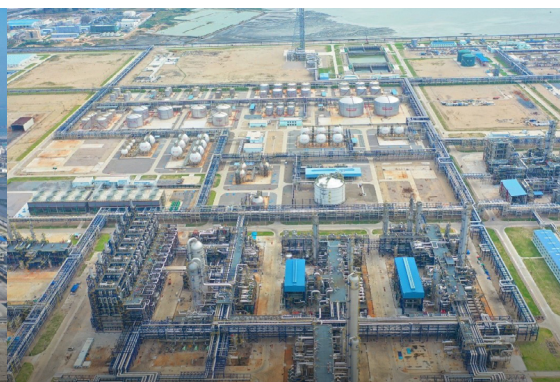
Aerial view of the steam cracking unit
