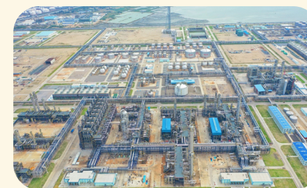
Aerial view of the steam cracking unit
