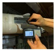
Chiller Water In/Out Temperature Measurement
